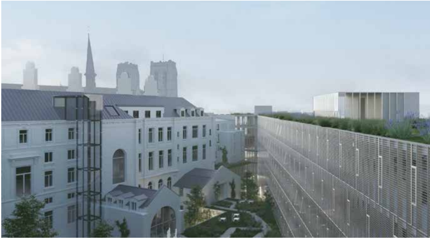
The new headquarters will be an energy-neutral and future-proof building designed in accordance with circular economy principles.
